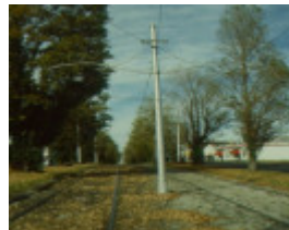
ornamental tramway overhead poles peel street
