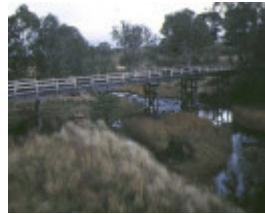
1 ellerslie bridge over hopkins river ellerslie side elevation
