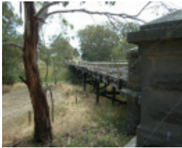
ELLERSLIE BRIDGE SOHE 2008
