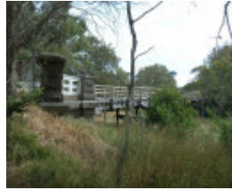
ELLERSLIE BRIDGE SOHE 2008
