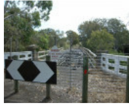
ELLERSLIE BRIDGE SOHE 2008
