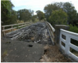
ELLERSLIE BRIDGE SOHE 2008
