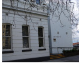
4679 Town Hall 1251 High Street Malvern Addition at Rear 1
