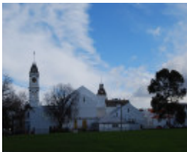
4679 Town Hall 1251 High Street Malvern Rear 1
