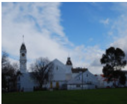
4679 Town Hall 1251 High Street Malvern Rear 1
