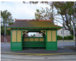
Tram Shelter Dandenong Rd Caulfield May 2006 North Side
