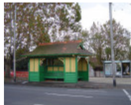
Tram Shelter Dandenong Rd Caulfield May 2006 South Side
