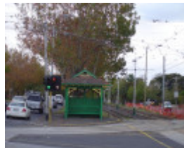
H0230 Tram shelter Dandenong Rd Caulfield May 2006 side view pj
