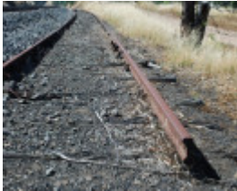
RAVENSWOOD RAILWAY SIDING SOHE 2008
