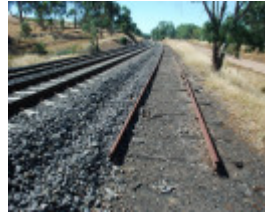
RAVENSWOOD RAILWAY SIDING SOHE 2008
