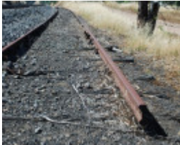
RAVENSWOOD RAILWAY SIDING SOHE 2008
