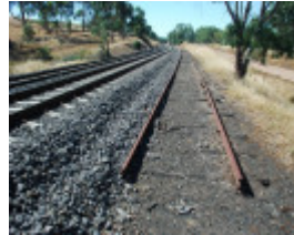
RAVENSWOOD RAILWAY SIDING SOHE 2008
