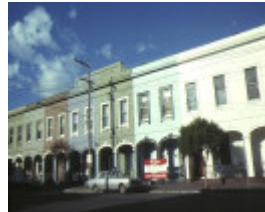
1 falconer terrace 36 napier street fitzroy mid section sep1978
