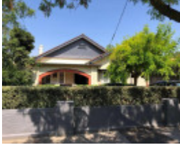
2 Devonshire Road, Malvern East
