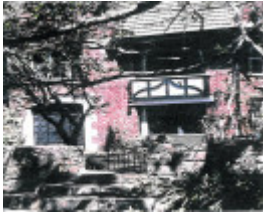
47485 House - Atkinson Street, Templestowe
