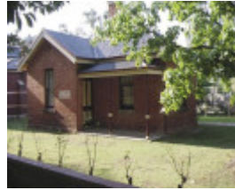
1 former lands office benalla front view mar1994
