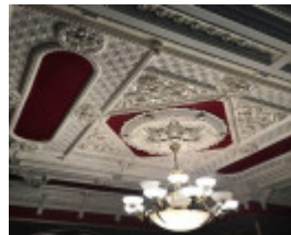
2019 gr floor sth east room ceiling.jpg
