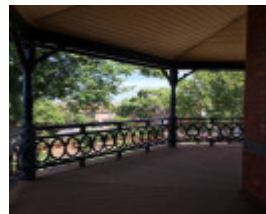
2019 first floor verandah.jpg
