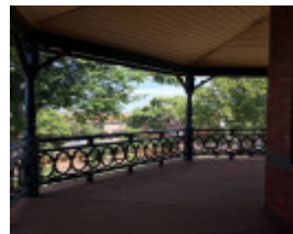
2019 first floor verandah.jpg
