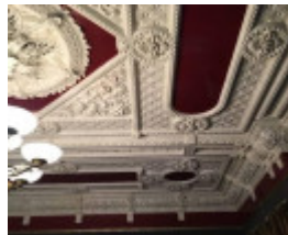
2019 gr floor sth east room .jpg
