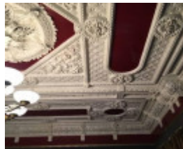
2019 gr floor sth east room .jpg
