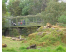
Lion enclosure prior to demolition 2014.jpg
