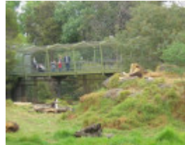
Lion enclosure prior to demolition 2014.jpg
