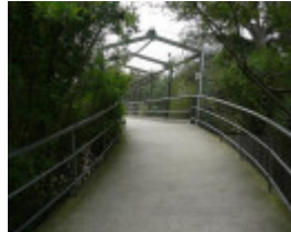
Lion enclosure prior to demolition, 2014.jpg
