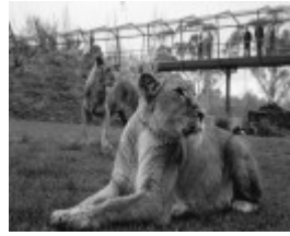
Lion enclosure prior to demolition 2014.jpg
