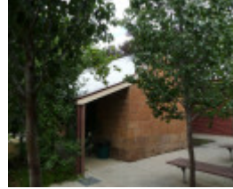
POLICE STATION AND OLD LOCK-UP SOHE 2008
