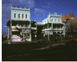
osborne house nicholson street fitzroy front view jun1979
