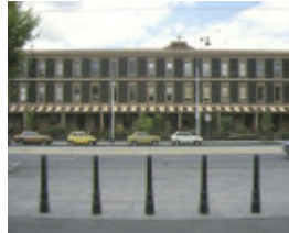
1 royal terrace nicholson street fitzroy front elevation feb1986
