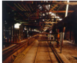
h01169 1 former donaghys ropeworks pakington street geelong finterior apr1997
