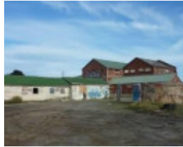
2013 Amenities building, main building and tanks from north east.jpg
