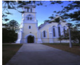
1 st george the martyr church & parish hall hobson street queenscliffe front view
