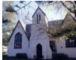
h01125 st george the martyr church and hall hobson st queenscliffe facade school hall she project 2003
