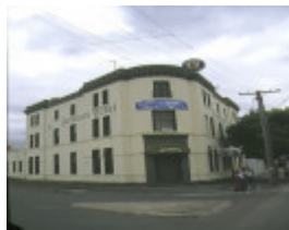
1 terminus hotel geelong front corner view apr1997
