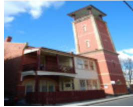
H0519 Fire Station 50 Macquarie St Prahran View South East 1 1
