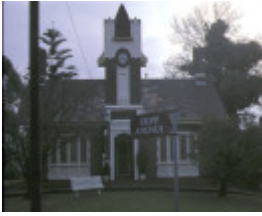
fripp avenue 9 fripp avenue front view aug1990
