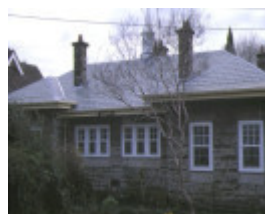
henty avenue & 7 henty avenue rear view aug1990
