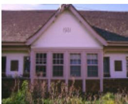
henty avenue & 5 henty avenue rear view aug1990
