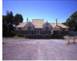
1 wonthaggi railway station front elevation jan1985
