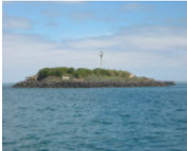
SOUTH CHANNEL FORT SOHE 2008
