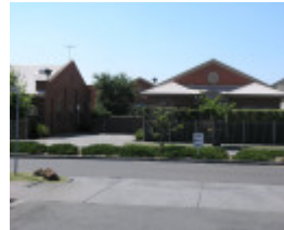
FORMER ROYAL AUSTRALIAN FIELD ARTILLERY BARRACKS SOHE 2008
