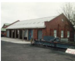
H01098 rafa barracks gun shed 1995
