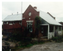
H01098 rafa barracks horse hospital demolished 1995
