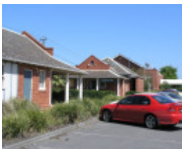
FORMER ROYAL AUSTRALIAN FIELD ARTILLERY BARRACKS SOHE 2008
