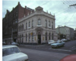
1 former union bank of australia smith street fitzroy corner view mar1980
