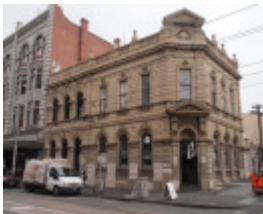
H0506 FORMER UNION BANK OF AUSTRALIA LHA 2015 1.JPG
