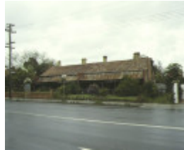
1 iron cottage brunswick road brunswick housing row 1992
