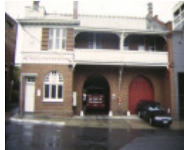
1 hawthorn fire station front view
