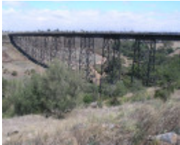
RAIL BRIDGE (ALBION VIADUCT) SOHE 2008
