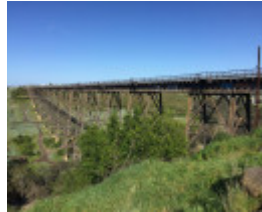
RAIL BRIDGE (ALBION VIADUCT) September 2016
