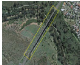
Albion Viaduct Extent Aerial June 2021
