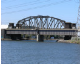
RAIL BRIDGE SOHE 2008
