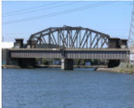
RAIL BRIDGE SOHE 2008
