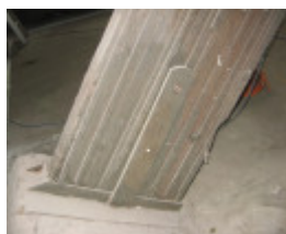
glue laminated beam abutment
