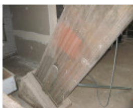
glue laminated beam abutment
