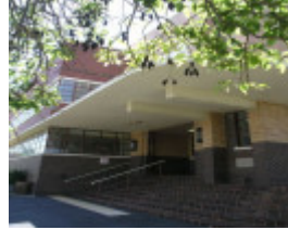
FORMER ESSENDON TECHNICAL SCHOOL SOHE 2008
