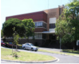
FORMER ESSENDON TECHNICAL SCHOOL SOHE 2008
