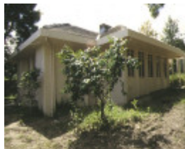
1 murray griffin house heidelberg side view dec1996
