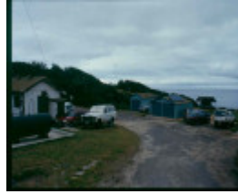
h01983 pt hicks generator shed dec99 pm1
