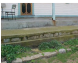
h01983 pt hicks asst qtrs verandah2 sep03 pm1
