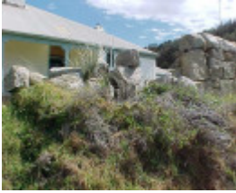
h01983 pt hicks drywall damage2 sep03 pm1
