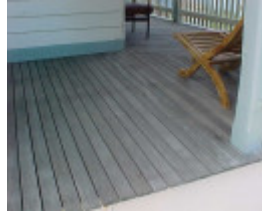
h01983 pt hicks verandah detail sep03 pm1
