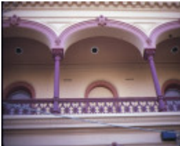
terrace 203 victoria parade fitzroy detail of balcony jul1984
