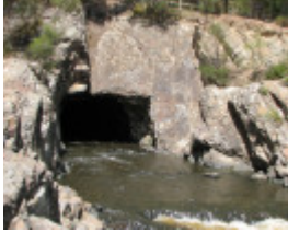
POUND BEND GOLD DIVERSION TUNNEL SOHE 2008
