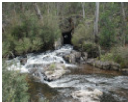
DELEGATE RIVER GOLD DIVERSION TUNNEL SOHE 2008
