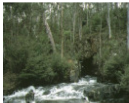
1 delegeate river gold diversion tunnel bonang entrance view
