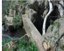
HOUGHTONS FLAT GOLD DIVERSION TUNNEL SOHE 2008
