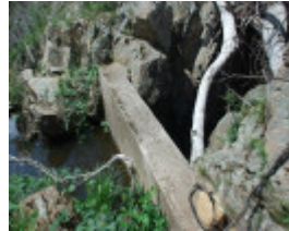
HOUGHTONS FLAT GOLD DIVERSION TUNNEL SOHE 2008
