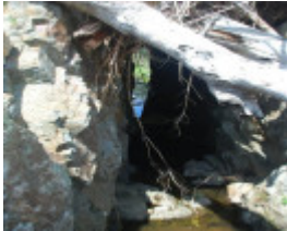
HOUGHTONS FLAT GOLD DIVERSION TUNNEL SOHE 2008
