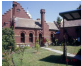
h01470 former flemington court house wellington street flemington garden she project 2004
