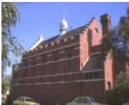
former flemington court house wellington street flemington side elevation may1987
