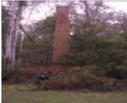
1 howqua united gold treatment works howqua hills track howqua front view
