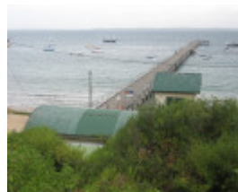
Jetty & shed - view from hill, Jan 2008
