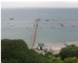
Jetty & surrounds - view from hill, Jan 2008
