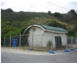
Former jetty cargo shed - view from south east, Jan 2008
