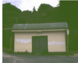
former jetty cargo shed flinders foreshore flinders front shed entrance
