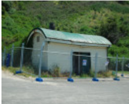
FORMER JETTY CARGO SHEDS SOHE 2008
