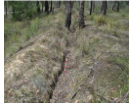
Water Race from Russels Reservoir (December 2019)
