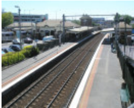
FOOTSCRAY RAILWAY STATION COMPLEX SOHE 2008
