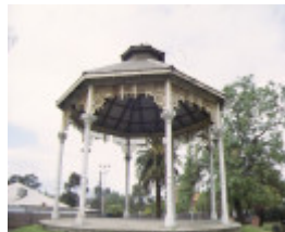
Footscray Railway Station Complex Irving Street Footscray Reserve Bandstand October 1998
