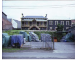
1 henderson house footscray front view
