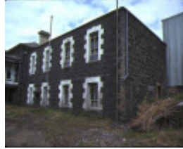
henderson house footscray bluestone building
