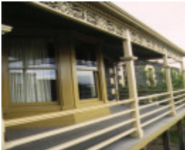
henderson house footscray verandah detail
