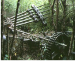
1 mount merrimac gold battery site lightning creek sunnyside front view
