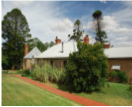
ADELAIDE VALE HOMESTEAD AND OUTBUILDINGS SOHE 2008
