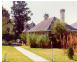
adelaide vale homestead and outbuildings goornong side view
