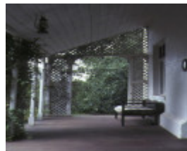
ballam park frankston front porch mar1984
