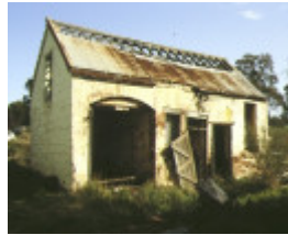
former leaky's residence millers road bacchus marsh stables aug1992
