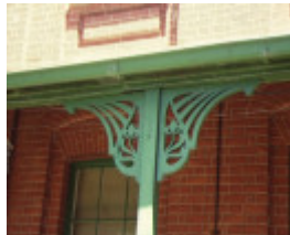
fulham park myrtlebank rd fulham detail verandah
