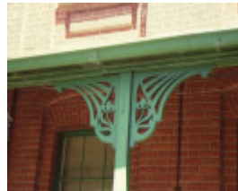
fulham park myrtlebank rd fulham detail verandah
