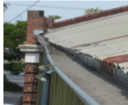
H1343 Existing condition - Eaves gutter north side. Dec 2006.
