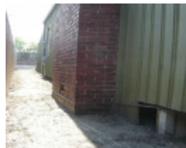
H1343 Exterior - South facade, with raised ground level. Dec 2006.
