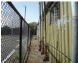
H1343 Exterior - West facade, with raised ground level. Dec. 2006.
