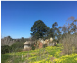
2019 outbuildings and Inn viewed from the north
