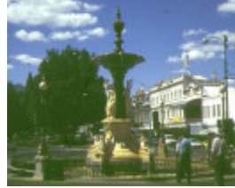
1 alexandra fountain bendigo front view mar1997
